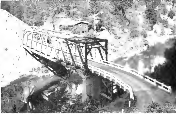
At left, old Salmon River Bridge at Somesbar, Siskiyou County. At right, how it looks rebuilt with steel salvaged from Eel River bridge at Scotia.
